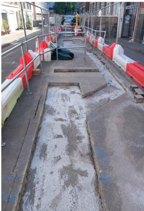
Euston Street Gas diversion – northern section backfilled
