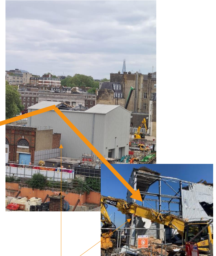
Removal of Acoustic shed progress above
