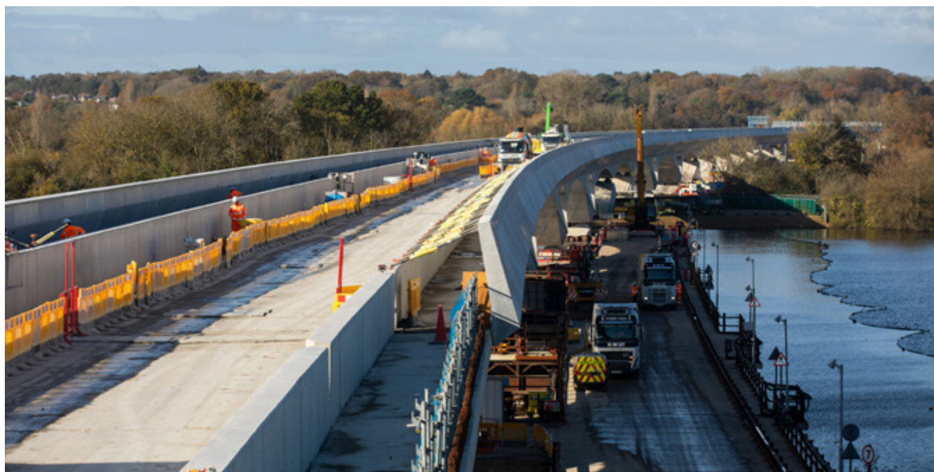
Robust kerb on the inside of the parapet walls as the viaduct crosses Harefield No2 lake, looking north, in November 2024.
