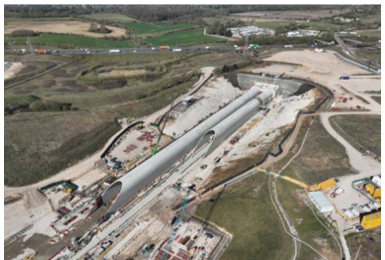
Chiltern tunnel south entrance showing two porous portal hoods.
