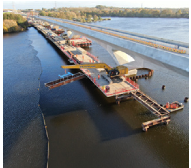
Long reach crane removing jetty on Harefield No2 lake.
