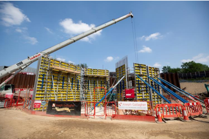
Upper level of reinforced concrete headhouse walls
