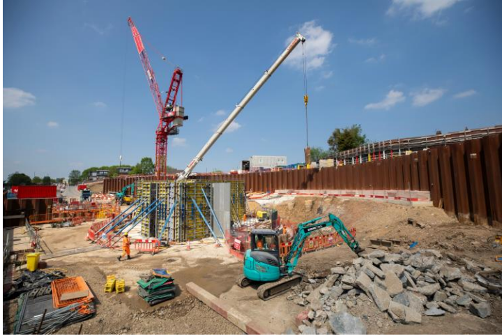
Lower level of reinforced concrete headhouse walls
