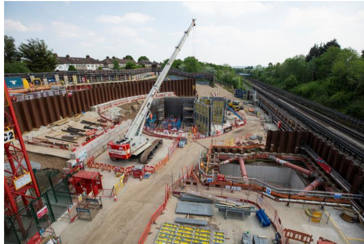
Aerial view showing ventilation basement and some headhouse walls
