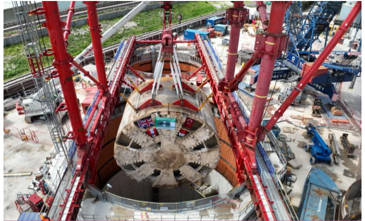
TBM Caroline lifted from Green Park Way vent shaft
