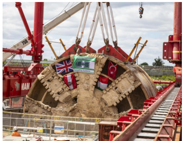
A close up of the extra-strong lifting attachments
