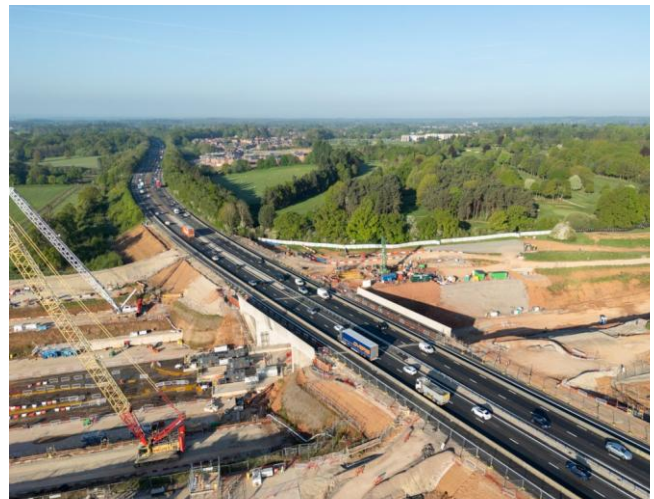
A46 box in position after the slide completion
