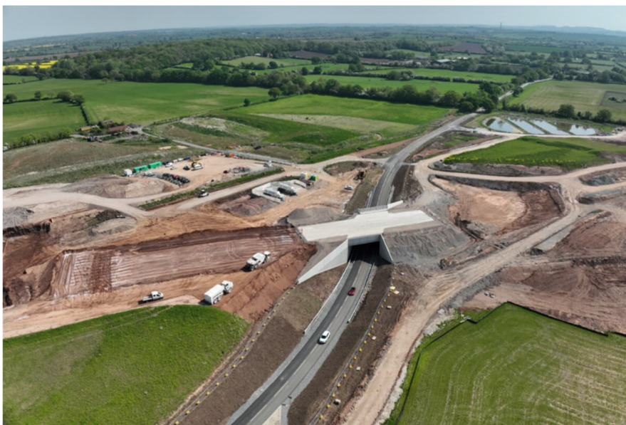
The Welsh Road Underbridge and realignment is now open
