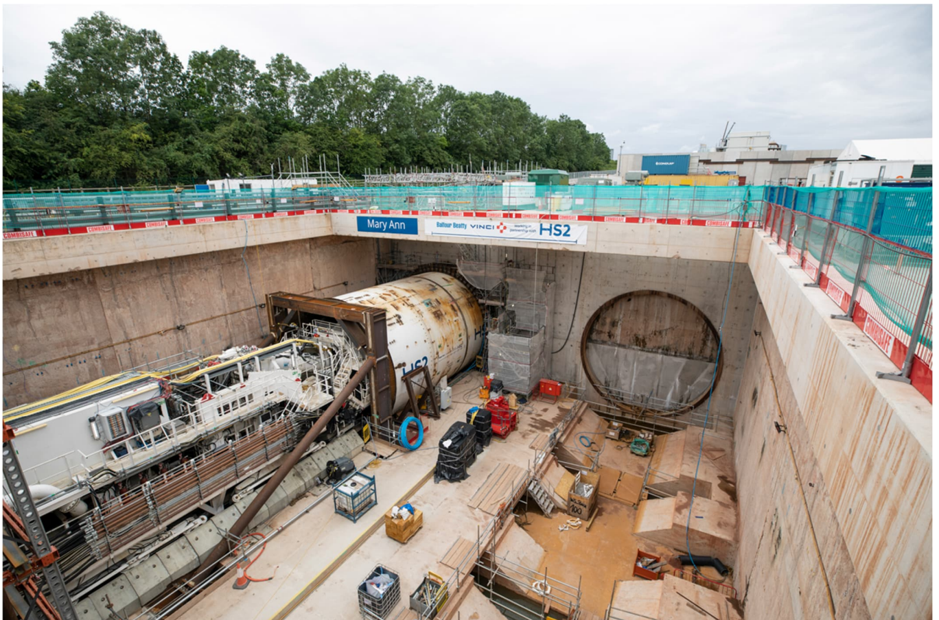
TBM Mary Ann at Bromford East Portal
