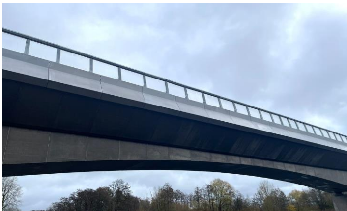
Noise barriers installed on top of the Colne Valley viaduct
