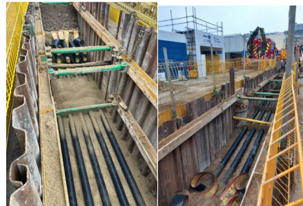
Photos of duct installation on Cobourg Street
