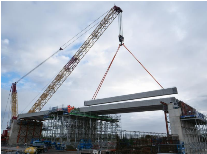
Figure 1: West Street overbridge beams being lifted into place, taken October 2024.
