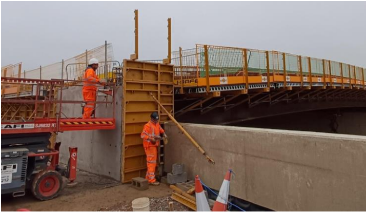
Figure 6: Stripping shutters from the diaphragms.
