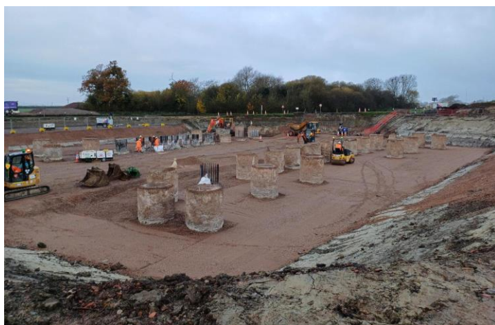
Figure 8: Pile cropping.
