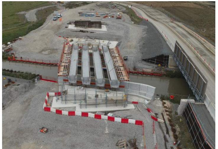
Figure 5: Deck beams installed over the Oxford Canal.
