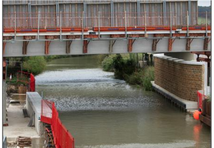
Figure 4: Stone cladding on the structure at canal level.
