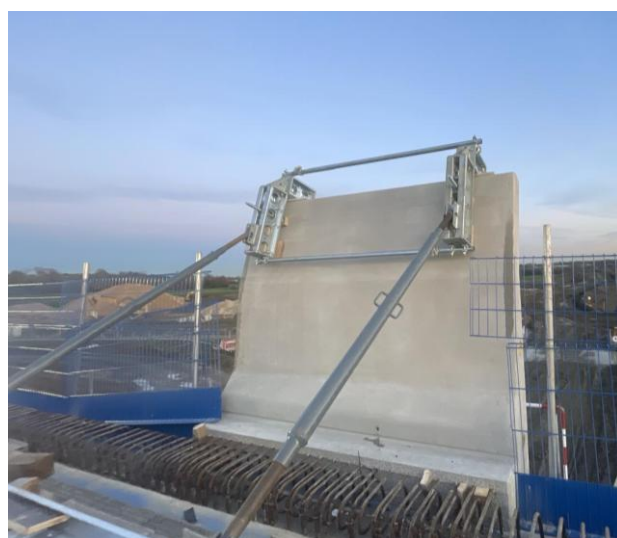
Figure 7: The first parapet was installed on Claydon Road overbridge in November.
