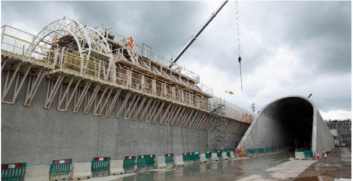
Porous portal construction at the South Portal site, in Hertfordshire.
