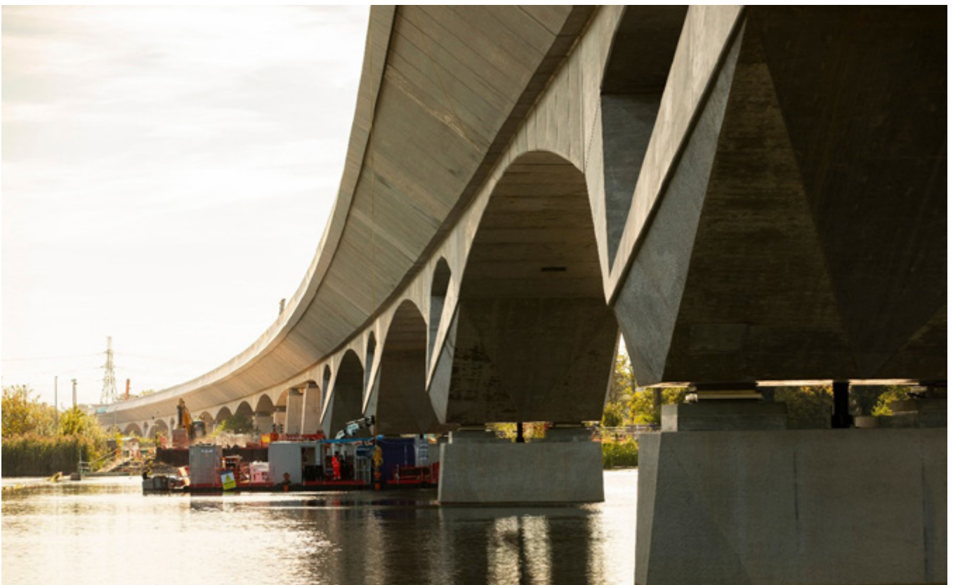
Piers in Korda Lake where the jetties and cofferdams used to create them are now being removed.
