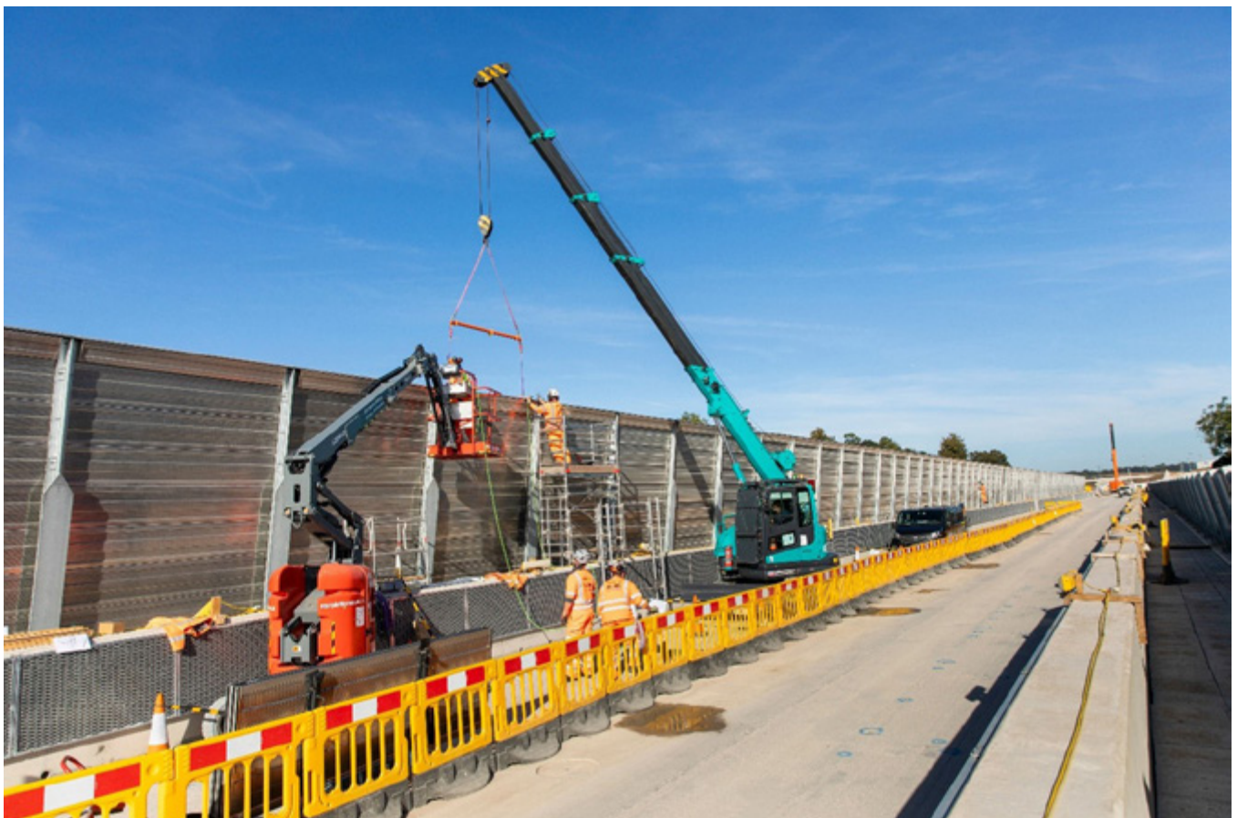
Four-metre-high noise barrier installation on the viaduct deck.
