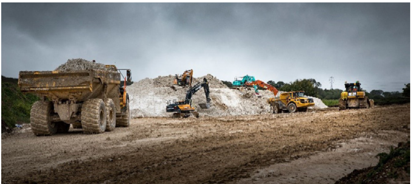
Earthworks to landscape the Western Slopes around the railway trace at the South Portal in Hertfordshire.
