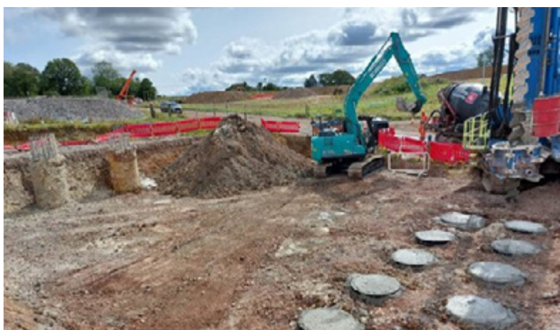
GMI/2 west platform after the completion of the piling works.
