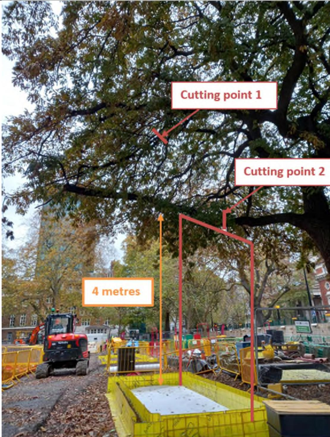
**Photograph No2:** Final Canopy position and proposed cutting point for the branches.
