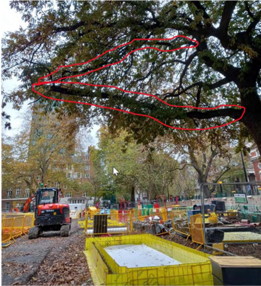
**Photograph No 1:** Illustrating view of the tree, indicating the branches that would collide with the canopy structure.
