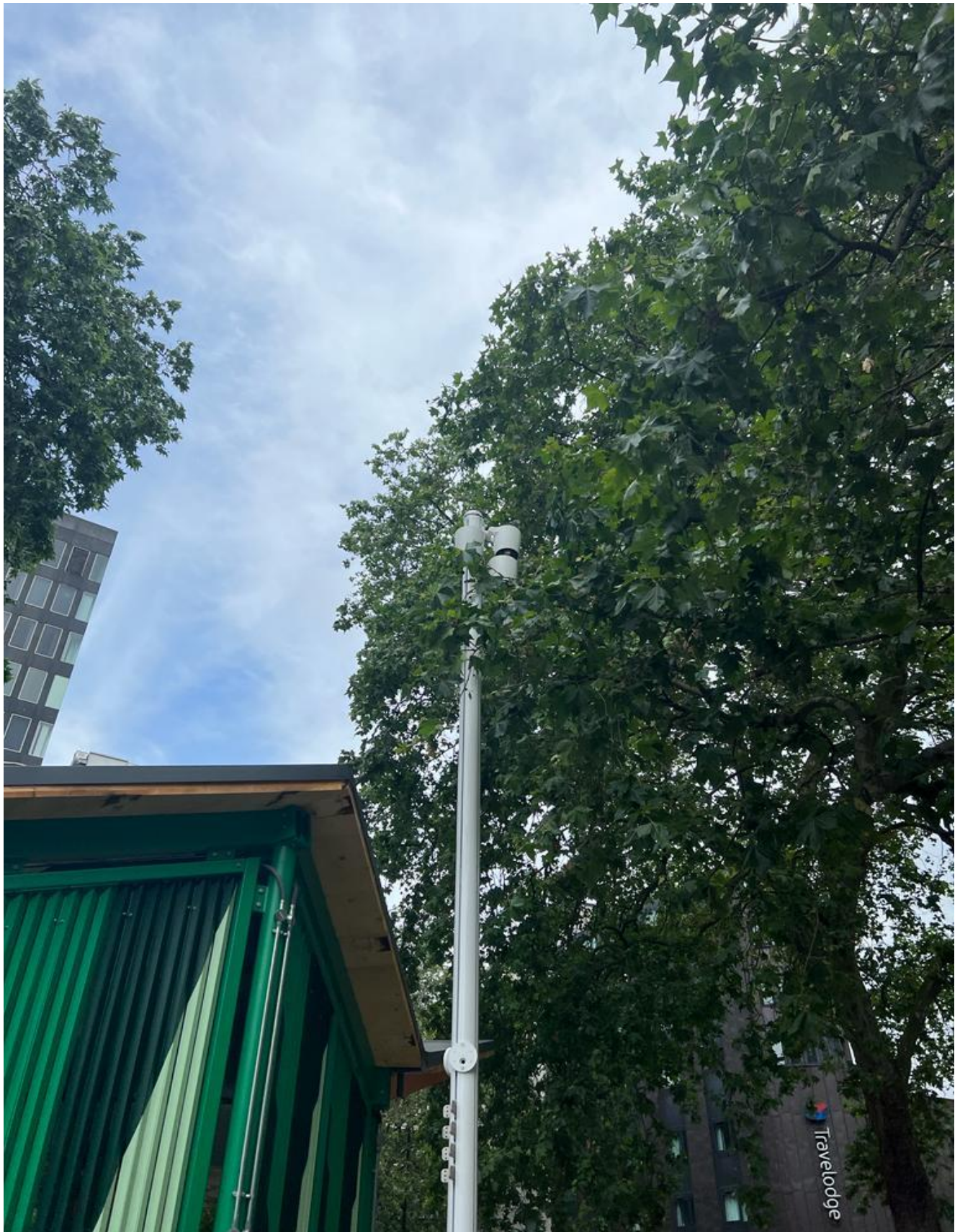
Photograph No 1: General overview of the lamppost with branches and foliage obstructing the lights on tree LP00862_T_F120.
