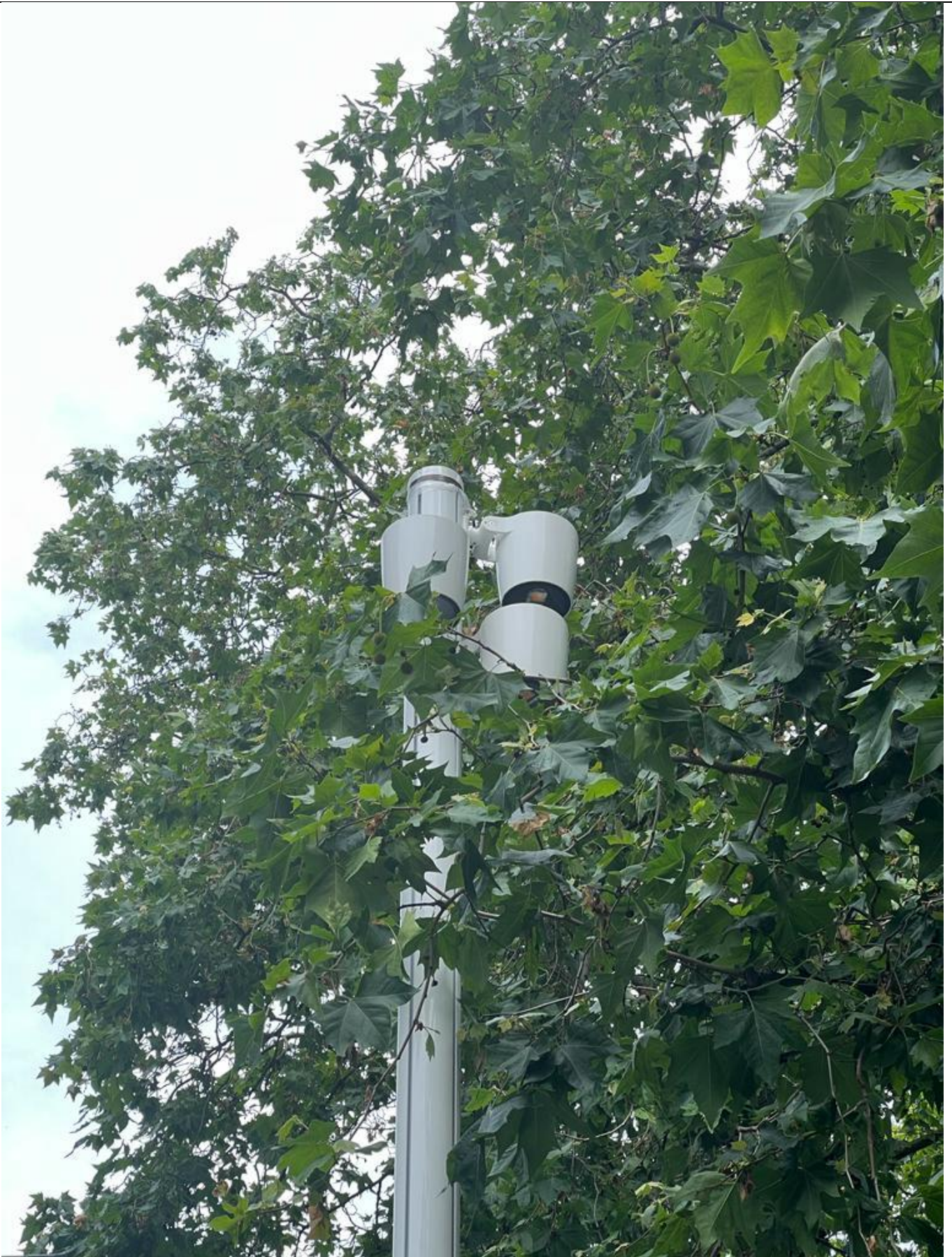
Photograph No 2: Zoom in view of the lamppost with branches and foliage obstructing the lights.
