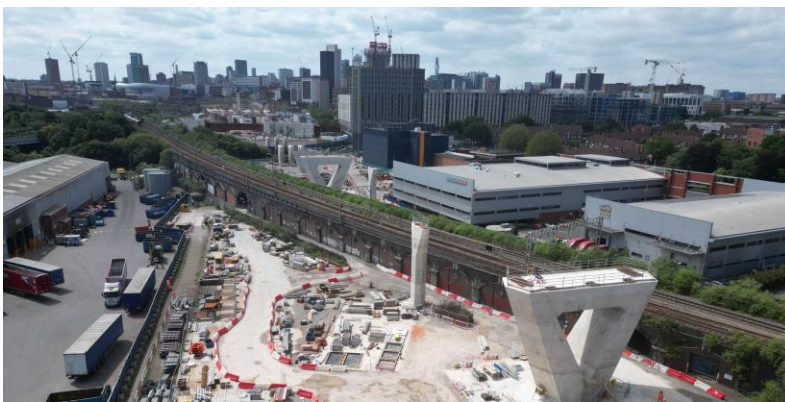
Curzon 2 viaduct piers either side of the existing railway
