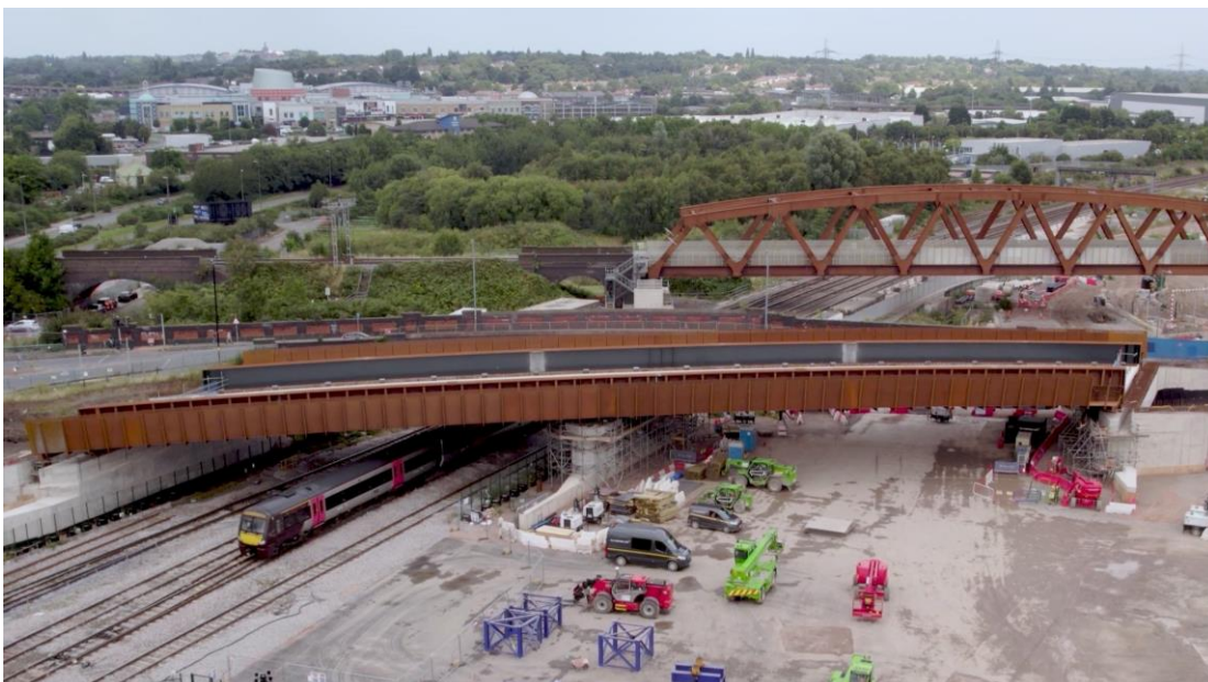
84 metre Aston Church Road bridge moved into place in five hours
