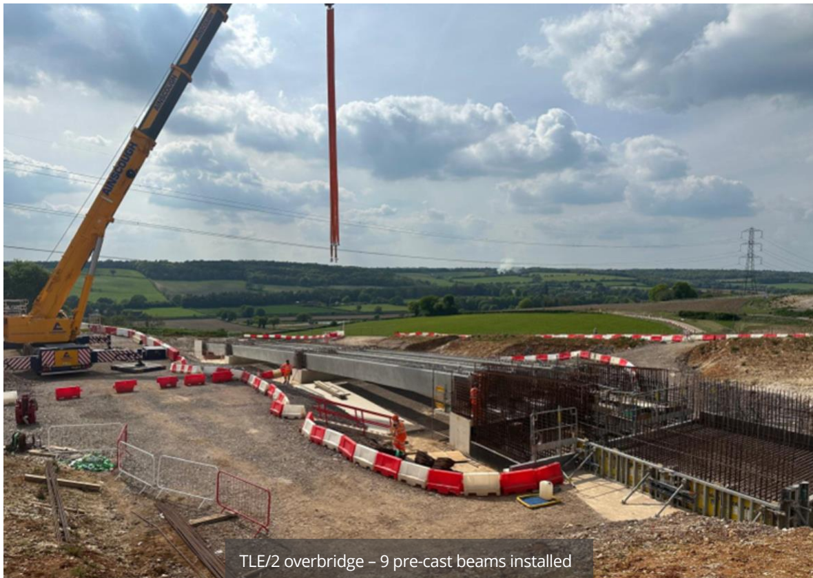
Construction of wing walls at Bowood Lane overbridge
