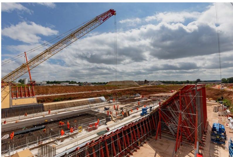
A46 Box construction showing base slab and bridge wall works (June 2024)
