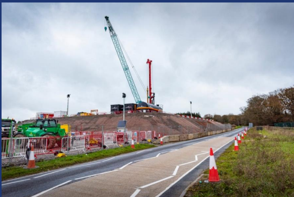
The newly constructed embankment at Rugby Road
