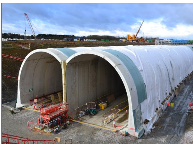
Chipping Warden green tunnel's waterproof membrane is being installed.
