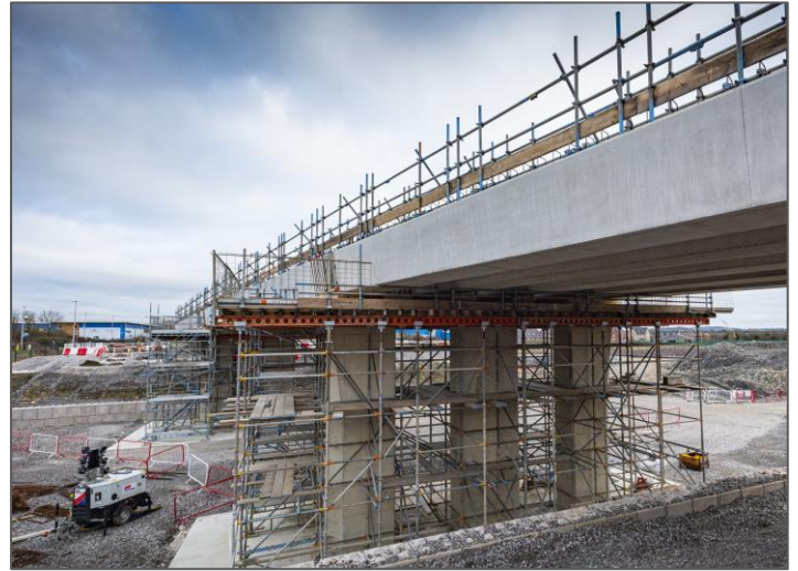
Bridge beams have been installed at Kineton Road
