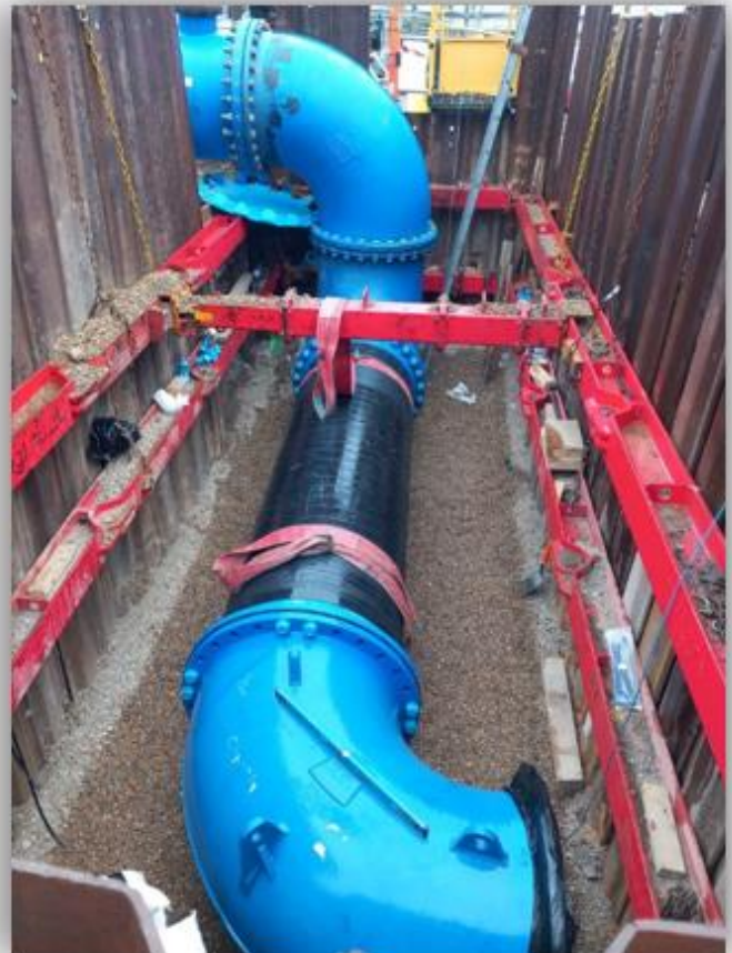
Image above on the right showing rider water bend installation on Cobourg Street and on the left - 1000mm water main rider installation on Cobourg St, south of Drummond St.
