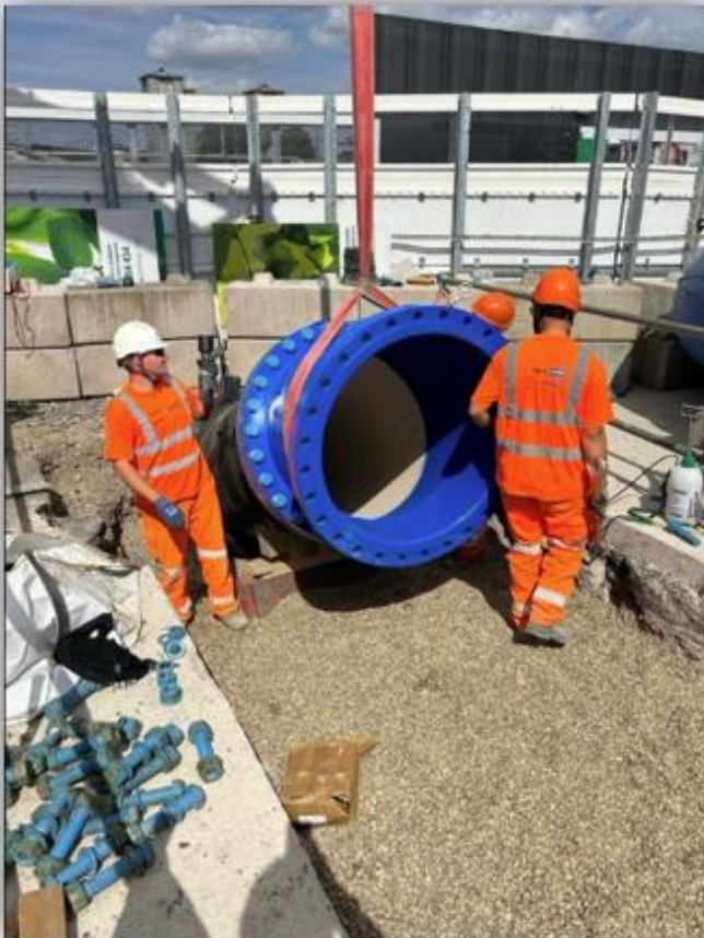
Image above on the right showing rider water bend installation on Cobourg Street and on the left - 1000mm water main rider installation on Cobourg St, south of Drummond St.
