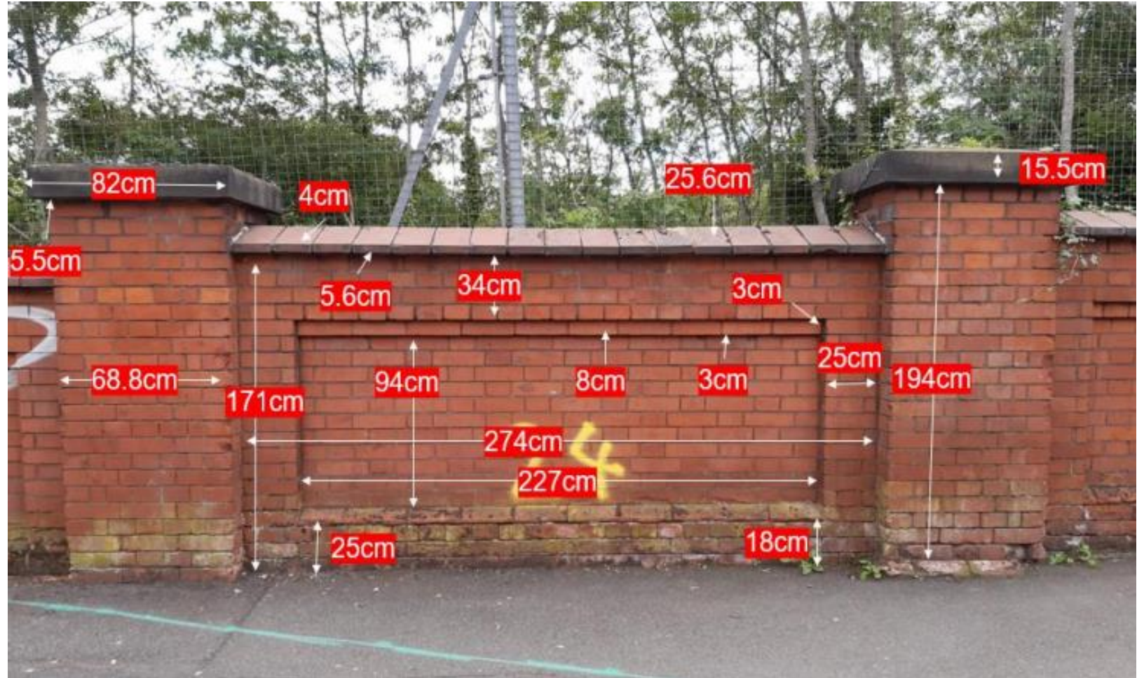
Annotated image taken from wall survey
