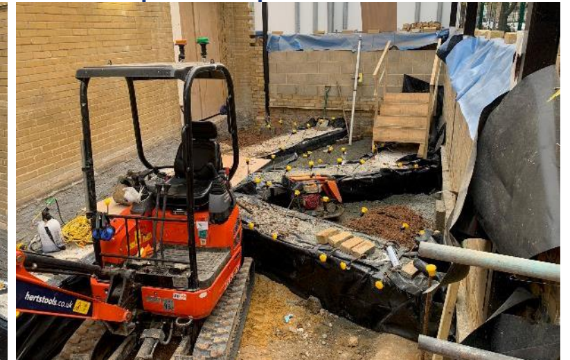
TEP Entrance Drainage and Thrust Block pours complete.
