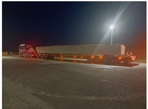
Thame Valley Viaduct beams being delivered
