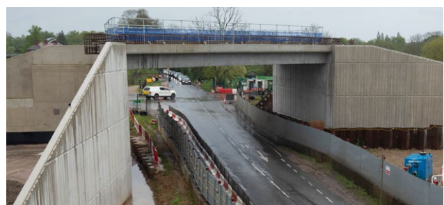
View of Breakspear Road South Underbridge looking from north - parapets not yet installed
