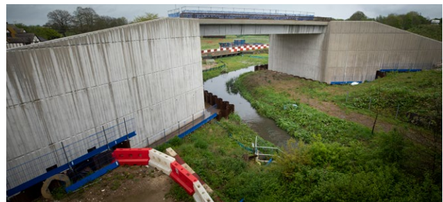
View of the River Pinn Underbridge from the south - parapets not yet installed
