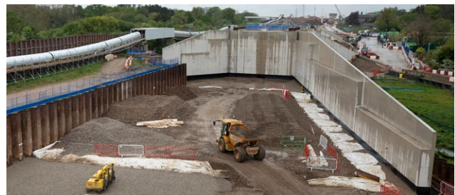
Embankment Construction works behind River Pinn Underbridge progressing with aggregate placement and compaction
