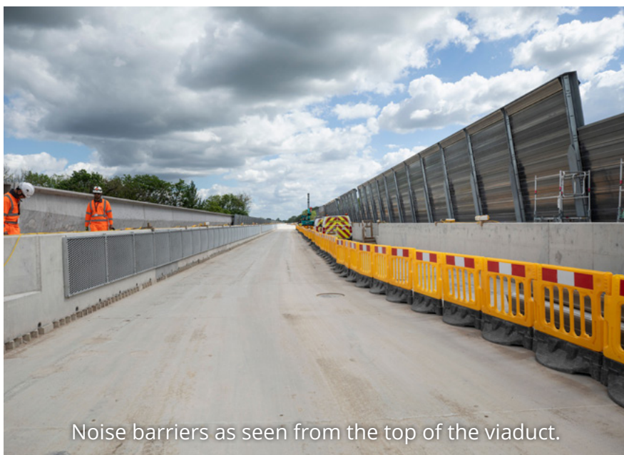
Noise barriers being installed on top of the Colne Valley viaduct
