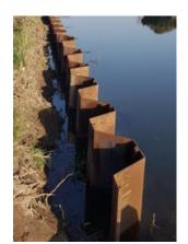
Sheet piling involves driving interlocking metal sheets into the ground, to create a strong retaining wall between the viaduct and the waterside.
