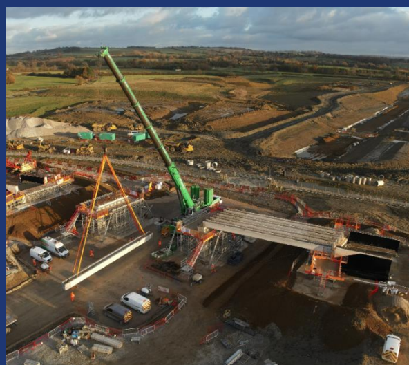
Lowering the deck beams into place in January 2024
