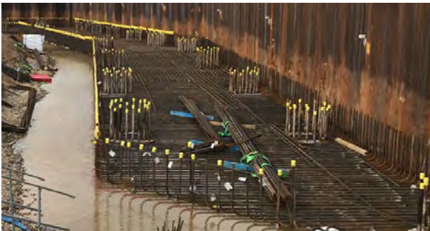
Steelworks on bridge structure on Harvil Road
