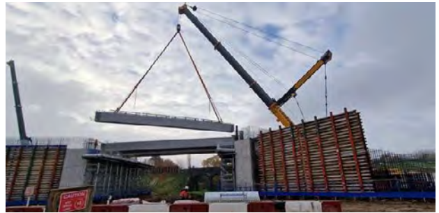
Concrete beam moved from Harvil Road to Breakspear Road bridge
