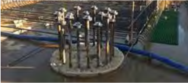
Steel fittings on foundations piles
