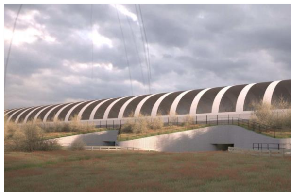
Figure 4: The computer-generated image above, is an artist's rendition of the south side of the Bat Protection Structure, showing the section which will include the Maxwell Brooke River culvert and the pedestrian footpath.
