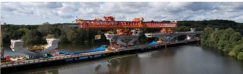
The launching girder installing sections of the viaduct deck between two piers.
