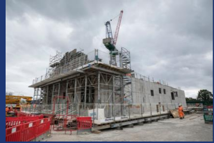
External walls erected at Chalfont St Peter headhouse.
