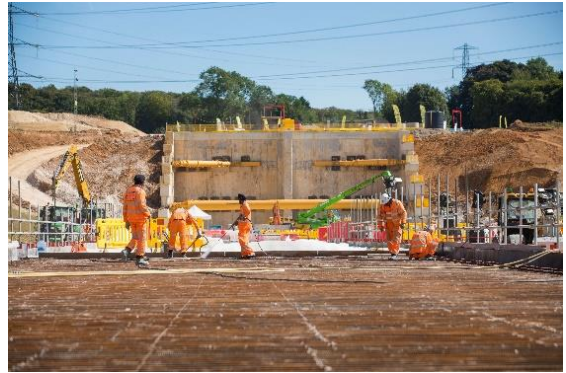
The North Portal head wall and track slab.
