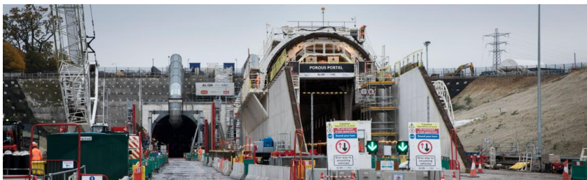
Works to create the Porous Portals at the Chiltern Tunnel South Portal site.
