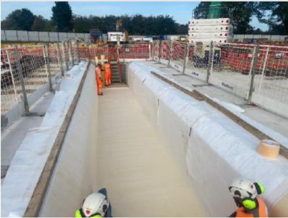
Headhouse trench waterproofing at Chesham Road.
