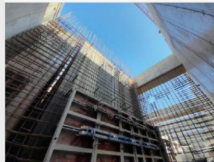
Steel fixing in Amersham basement.
