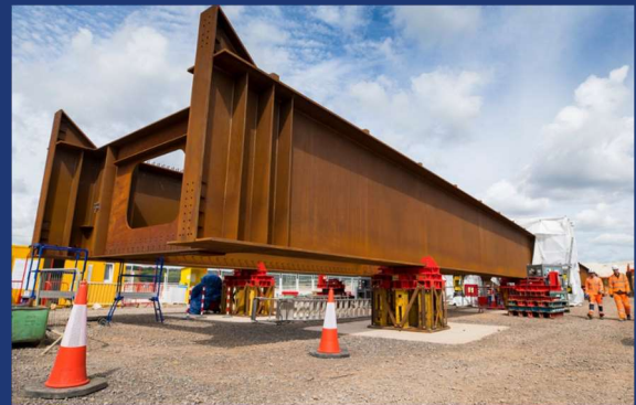
Steel works being positioned for the Wendover Dean viaduct.
