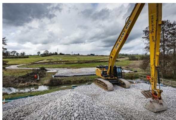
Figure 3: The T2G construction team lays the groundwork for a temporary bridge over the Great River Ouse, enabling us to efficiently move our internal construction traffic along our internal site access road.
