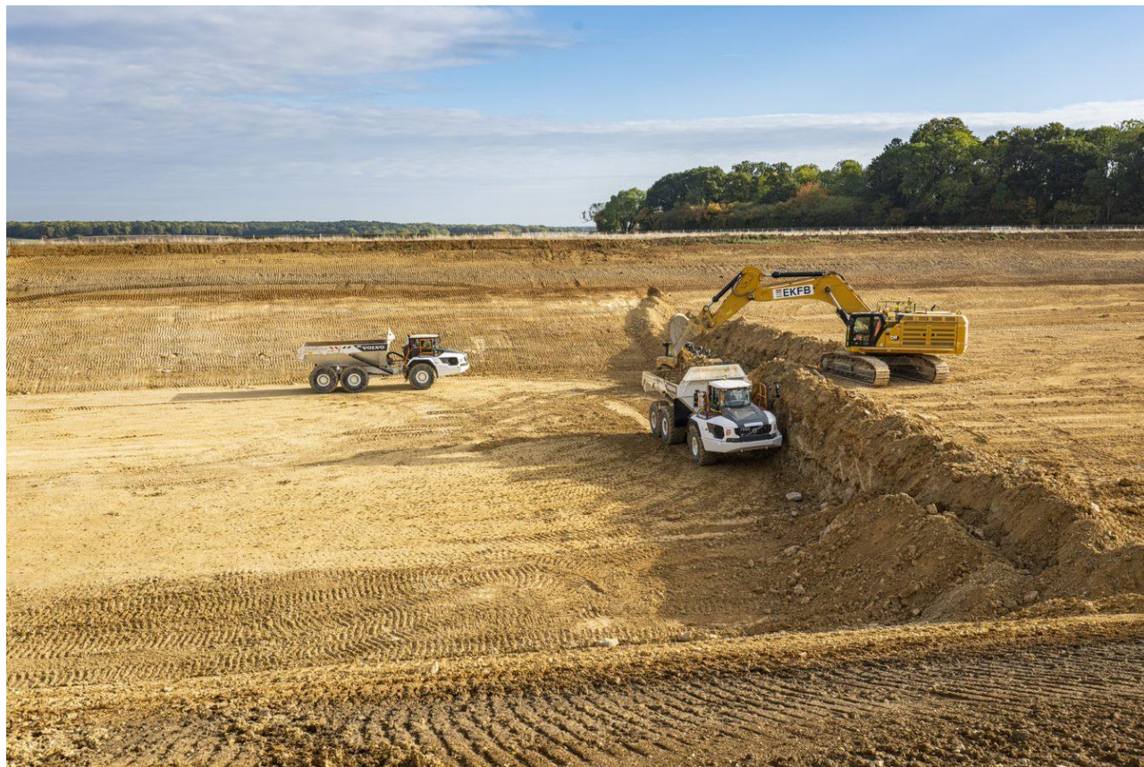
Figure 5: The image above is from one of our cuttings and shows how our teams carry out excavation works using large hydraulic diggers.
