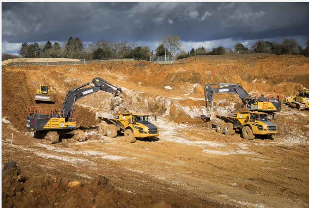
Figure 4: The image above shows machinery carrying out excavations for the South Heath Cutting in the North Chilterns Area, 2022.
