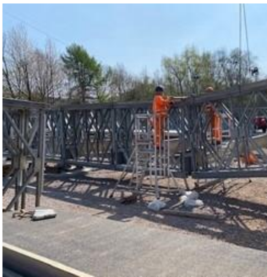
Figure 3: In the image above, you can see our teams working to install the 'Mabey Bridge' in April 2022.
