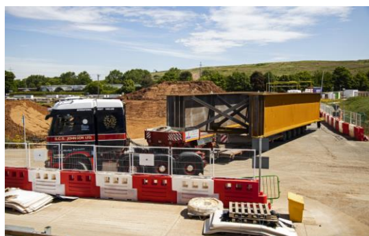
Figure 6: The above image is an example of an abnormal load of steel girders being delivered to an HS2 site.
