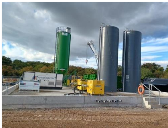
The image above shows the Bentonite Plant as it was being set-up in September at Small Dean Viaduct Launch compound.
