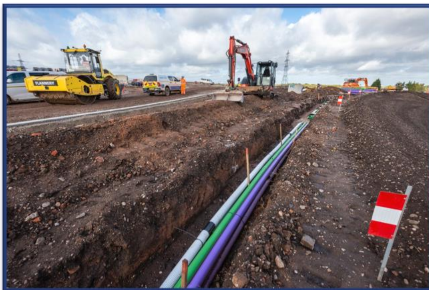
Utilities diversion are a key part of the construction process
