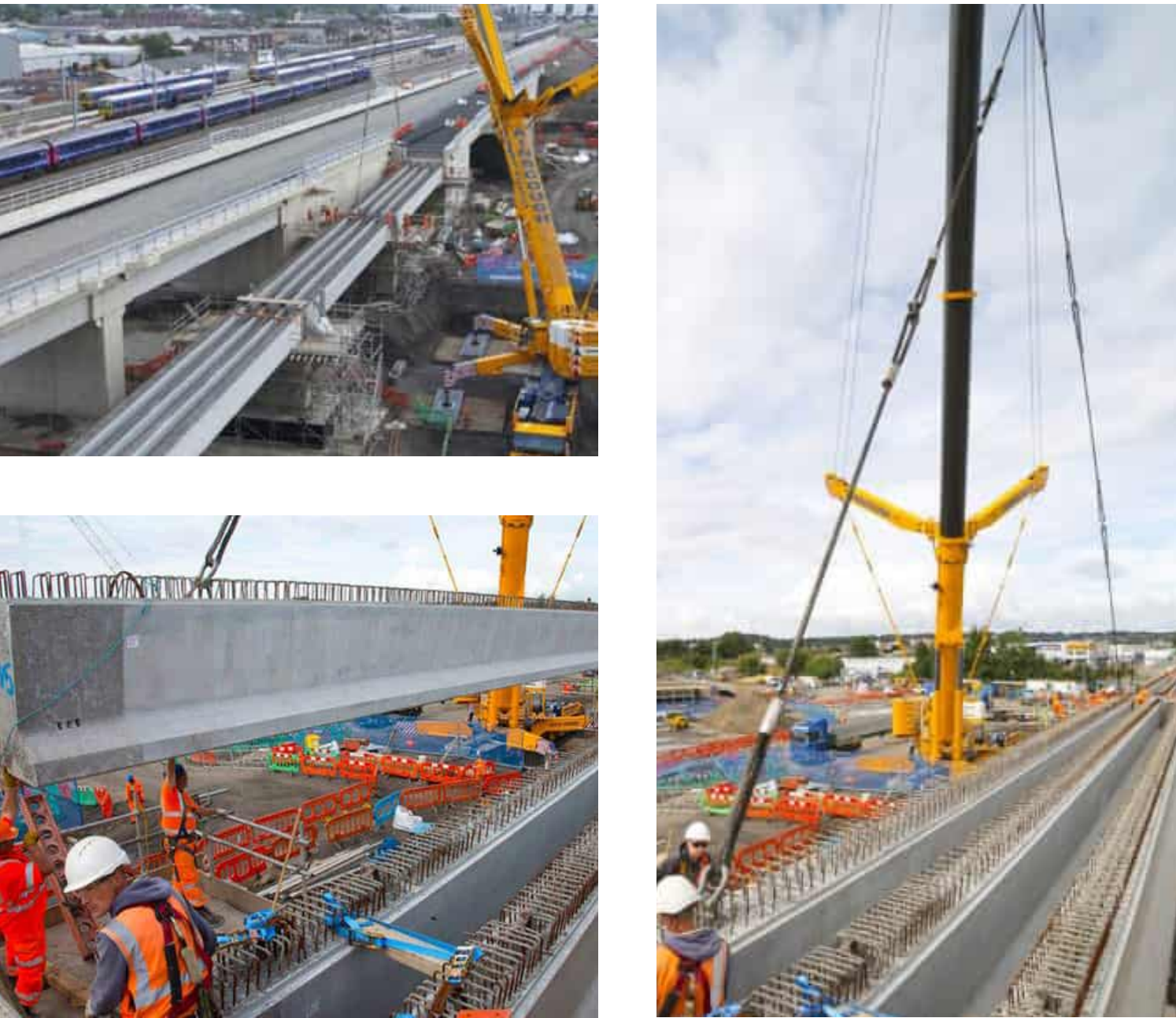
Photographs showing typical viaduct construction processes
