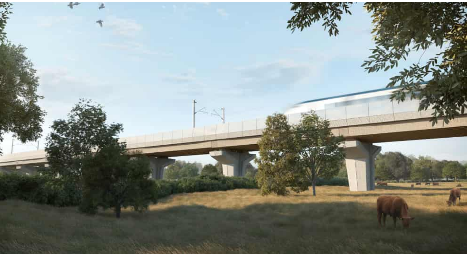
View from North side of Patrick Farm looking south
