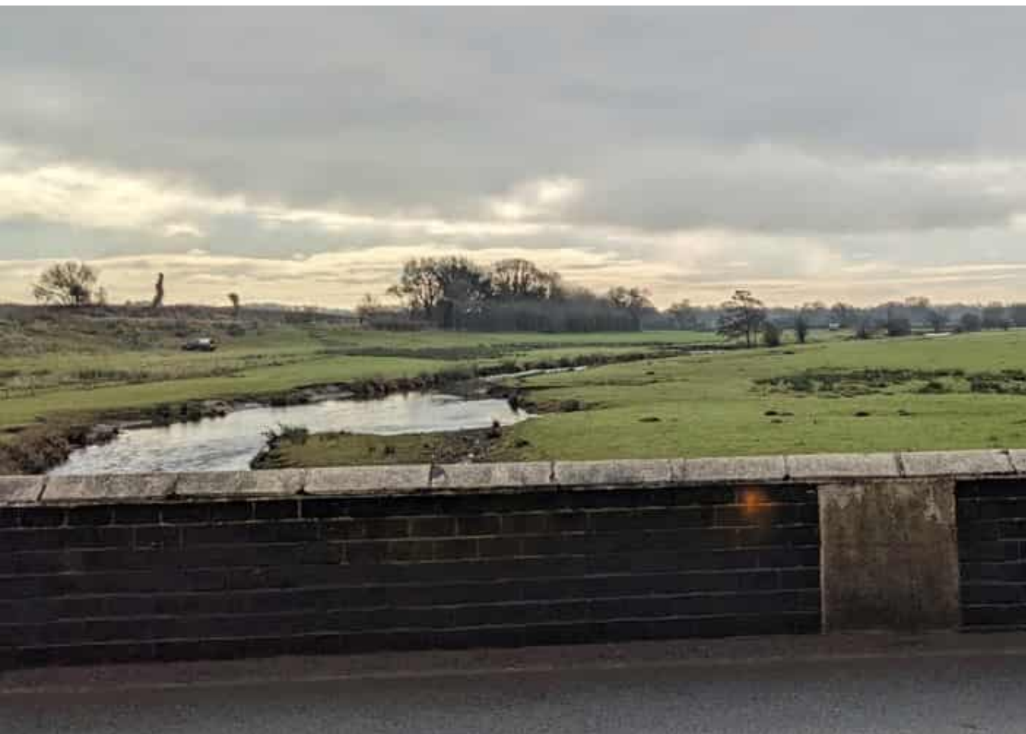
View A - from Patrick Bridge looking south-east
