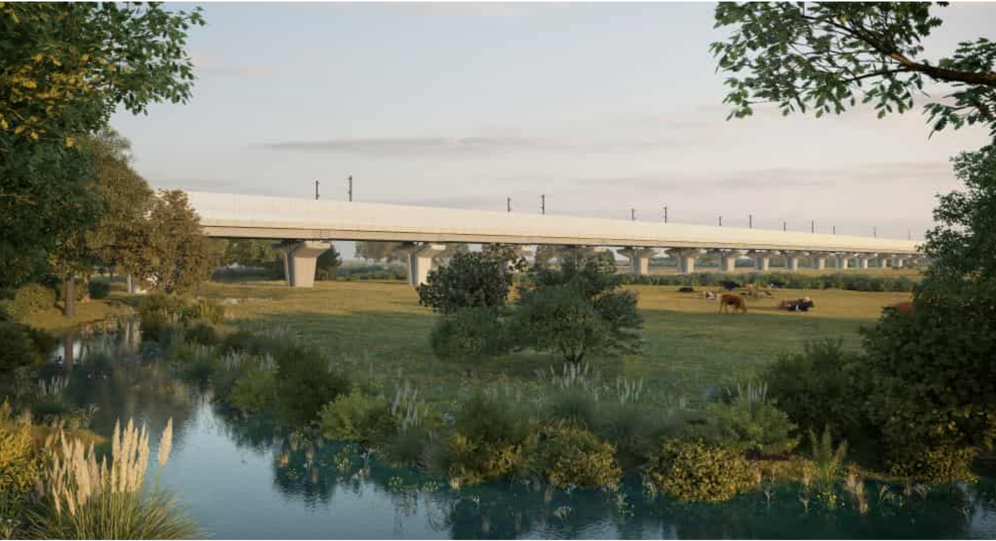
View from the River Blythe looking east
