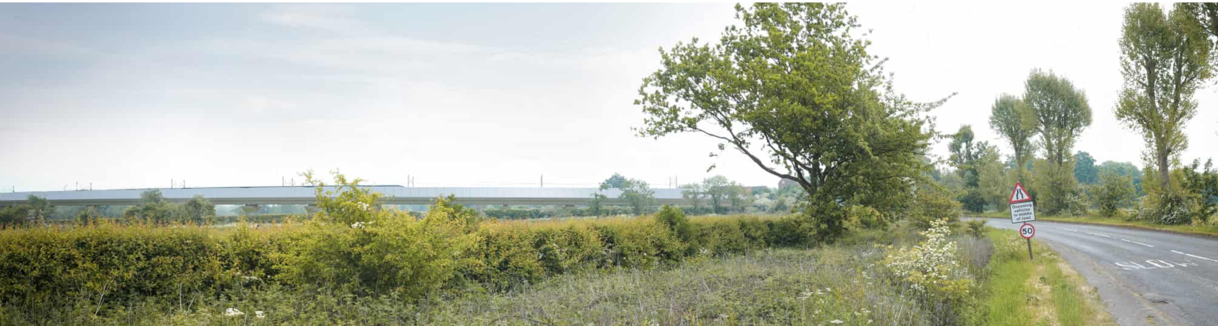
View from Meriden Road looking east
