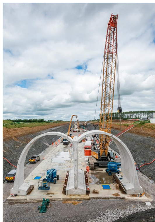
The tunnel is made up of 5 segments creating the double arch sections, this is repeated to create the 1.5 mile long green tunnel
