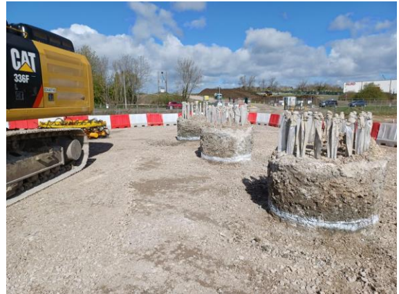
Once the concrete foundation piles are poured, the tops are capped off ready to support the structure.
