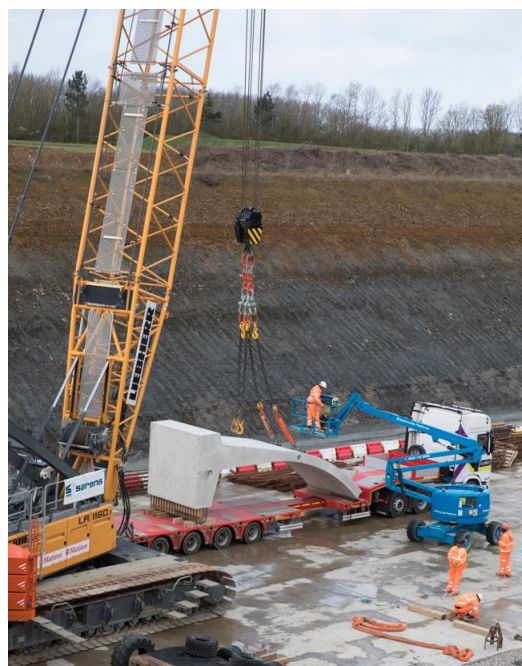
Pre-case tunnel segments will be coming into the Greatworth site on lorries, via approved routes, before being lifted into place using cranes.
