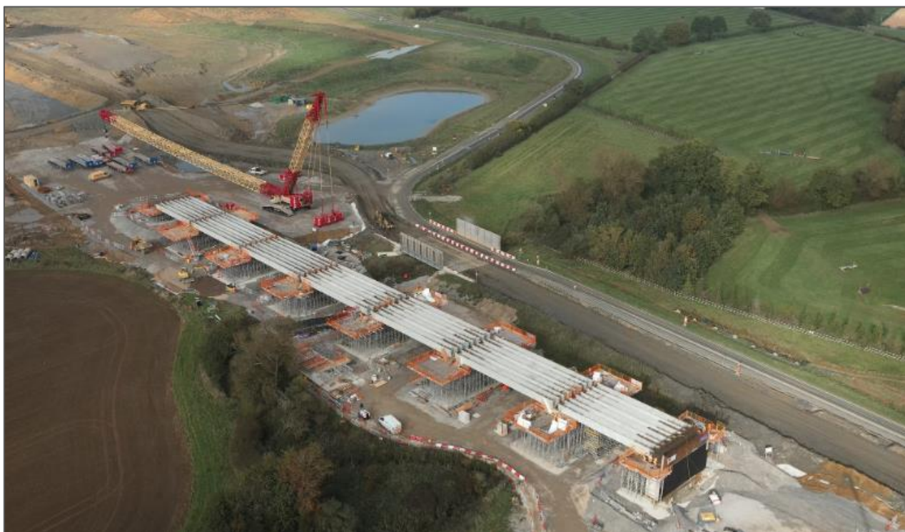
Aerial view of the beam installation and the 600 tonne crane that was used to lift the beams into place. This is the second viaduct on the HS2 programme to have all its beams laid.
