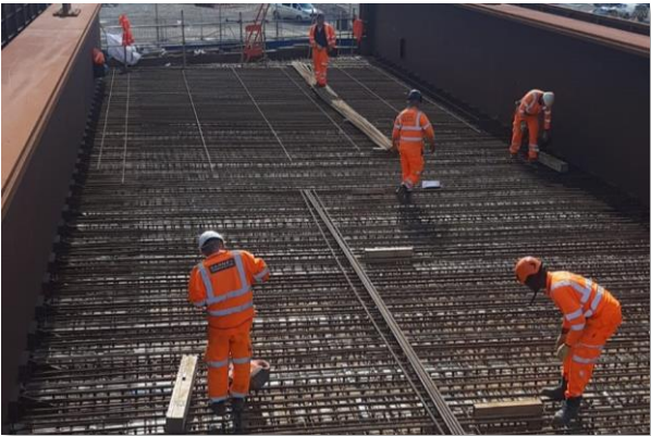
Rebar fixing works at the East West Rail overbridge deck
