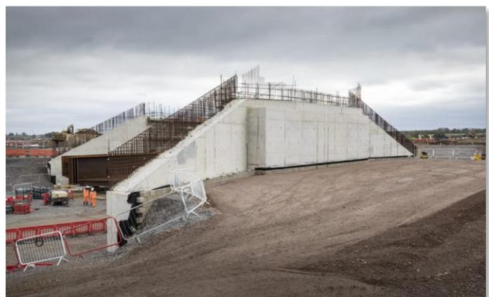
*Figure 3 : The image above shows the abutments and wing walls for the East West Rail Overbridge.*
