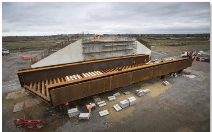
*Figure 3: The image above shows the assembled steel deck in preparation of the superlift, carried out in early December 2022.*
