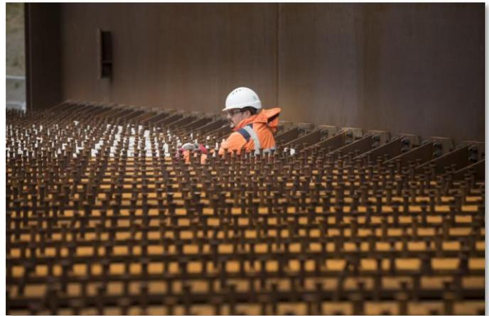
*Figure 3: The image above shows preparations taking place for the concrete element of the composite deck for the East West Rail Overbridge, November 2022.*
