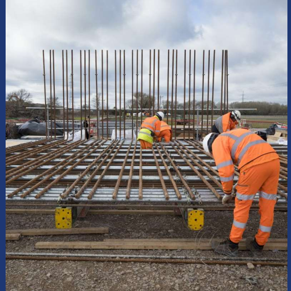
Steel frames being constructed ahead of concrete pouring on the PRA works.
