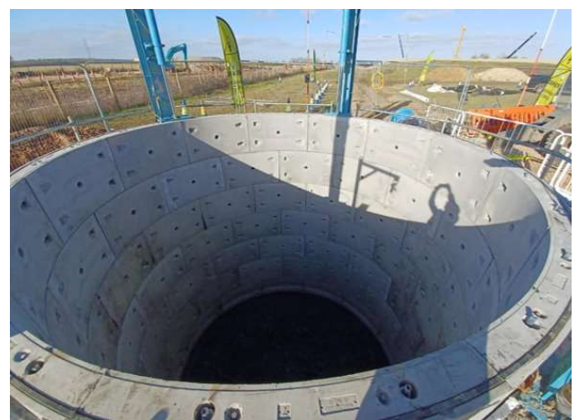
Auger bore shaft at the PRA
