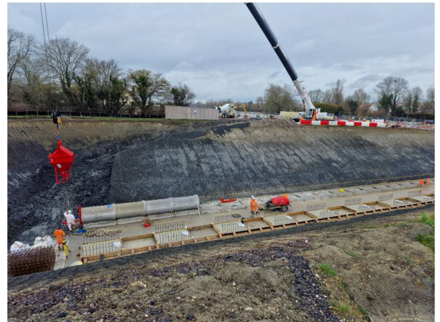
Pipe placing for the Thames Water sleeve at Risborough Road
