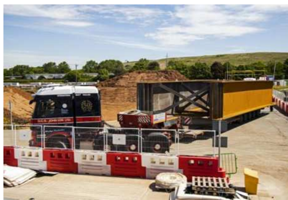
Figure 1: The above image is an example of an abnormal load of steel girders being delivered to an HS2 site.
