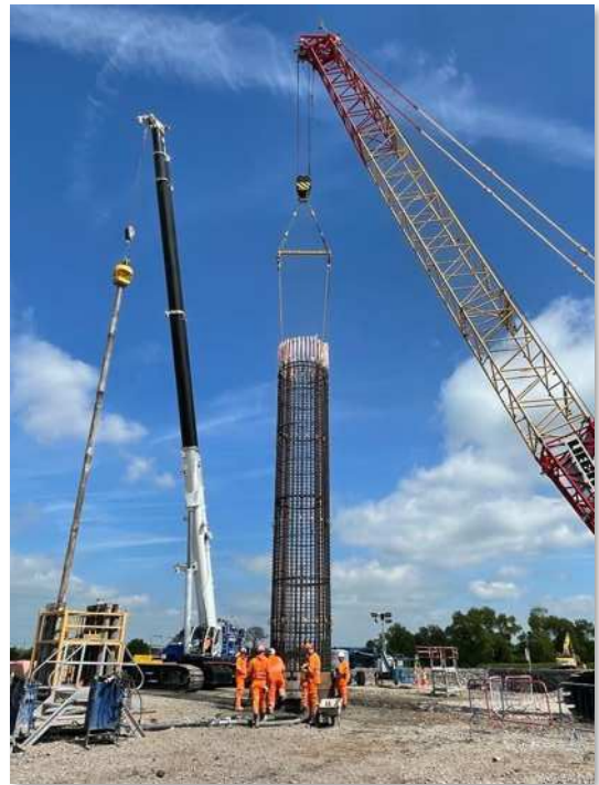
Figure 3: The above image shows our teams installing the first of four piers for the PRA overbridge.
