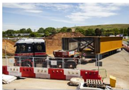
Figure 6: The above image is an example of an abnormal load of steel girders being delivered to an HS2 site.
