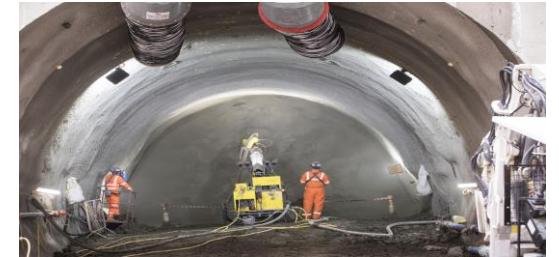
Step 2: Installation of primary sprayed concrete at the start of a tunnel
