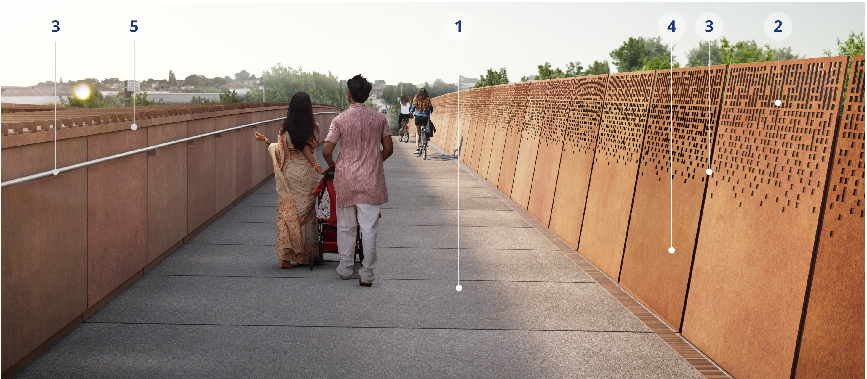
Final design: Saltley Viaduct walkway view showing warmer weathering steel balustrade
