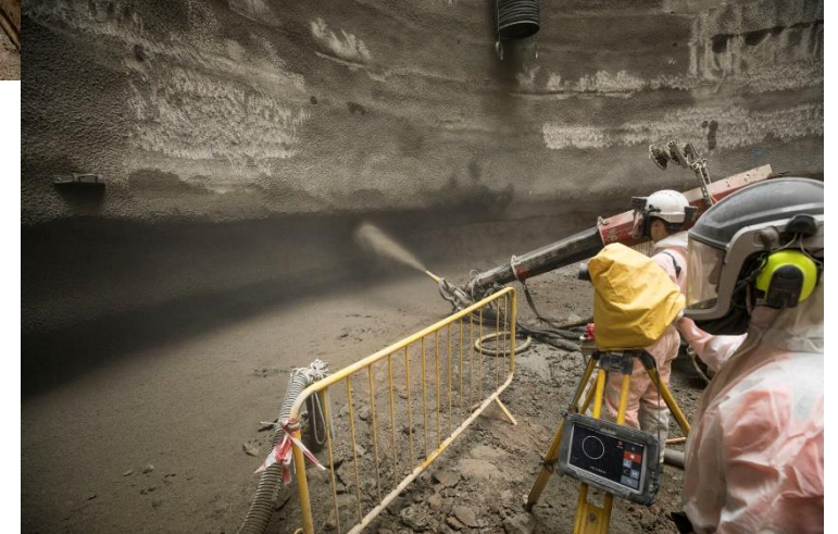
Examples of sprayed concrete lining (SCL) tunnelling
