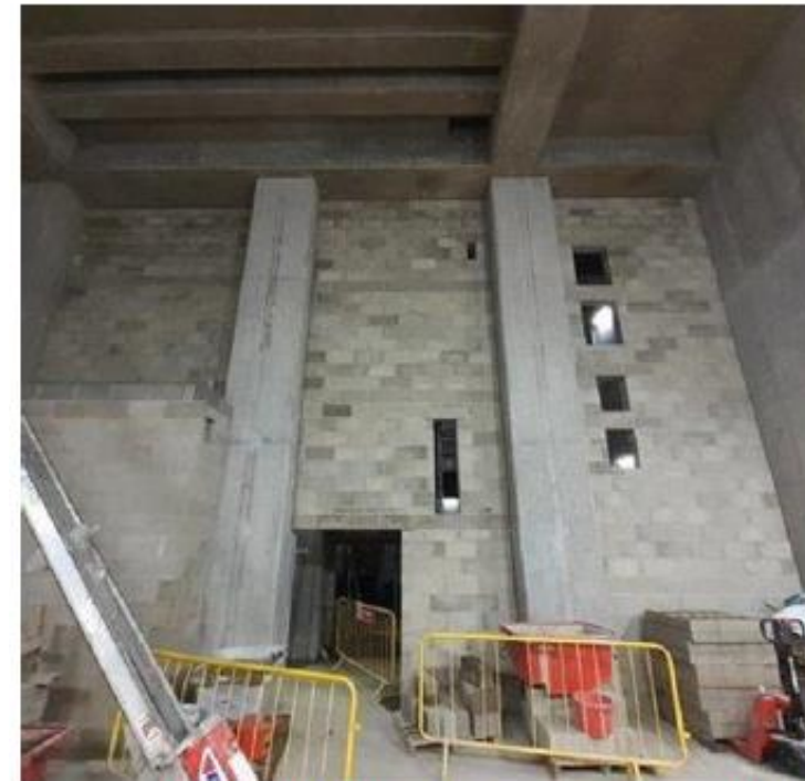
Basement level 3 blockworks up to 9 meters. April 2023
